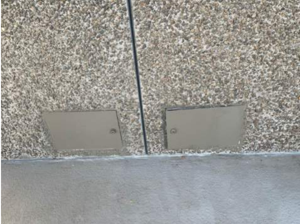
Figure 1: Painted access panels
