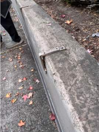
Figure 2: Site walls to be painted
