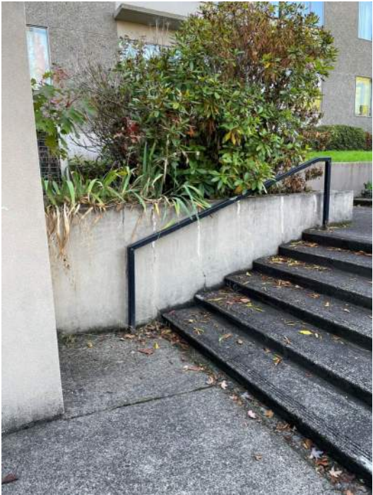
Figure 3: Site walls and handrails to be painted
