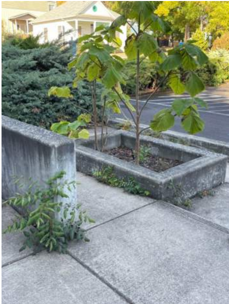
Unpainted site walls and planters to be pressure washed only
