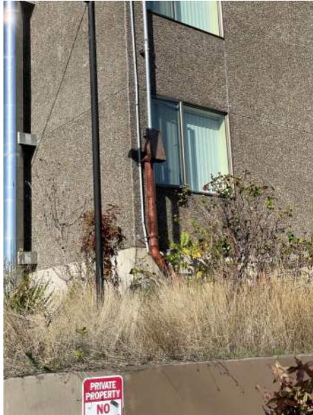
Paint out vented pipe and hood
