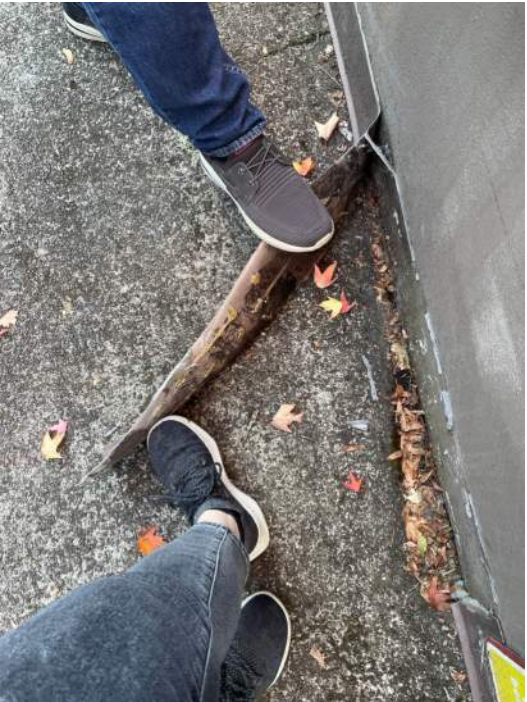
Figure 4: Remove rubber wall base on site walls
