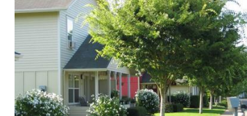
Walnut Park 32 Units Built 1995
