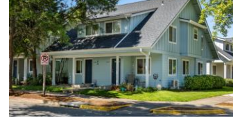
Jacob's Lane 63 Units Built 1998
