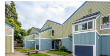
Pengra Court 22 Units Built 1980
