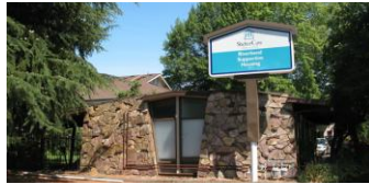
Signpost House 16 Units Built 2001
